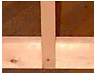
fig. 3: bottom brace with chiseled center support recess
